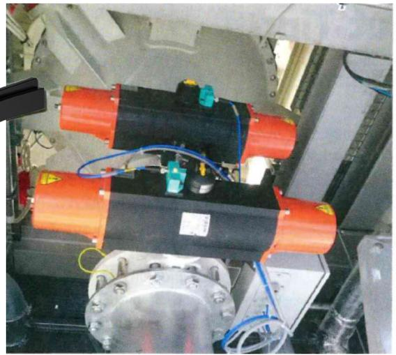
Fig. 3: The *clogged airlock* can generally be integrated in existing systems because of its lightweight and compact shape, without having to install complicated support structures or additional electrical supply lines.
